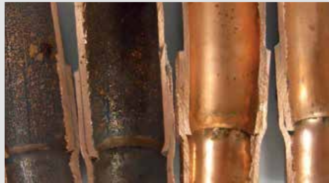
Without nitrogen purge
